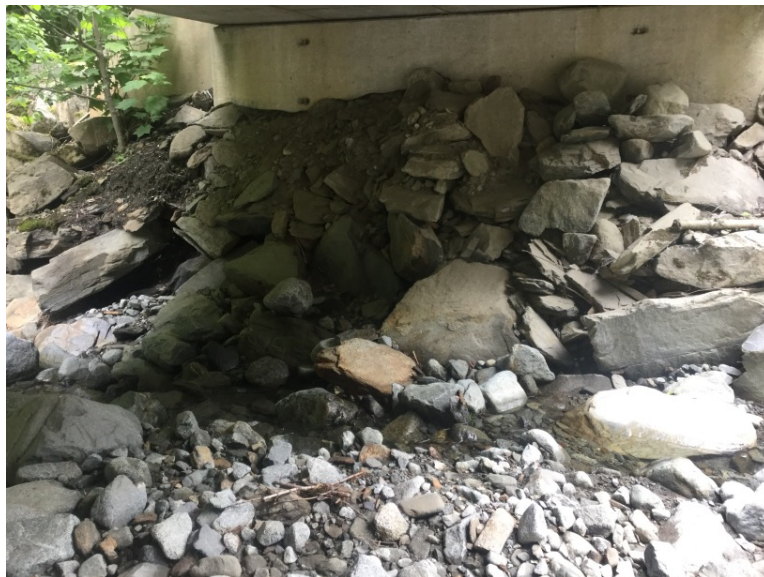
Right Bank Abutment when facing downstream
