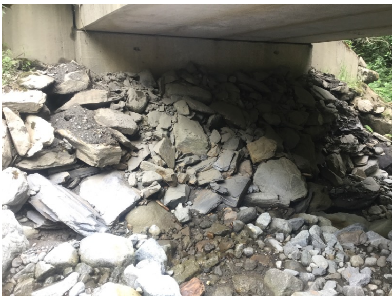
Left Bank Abutment when facing downstream
