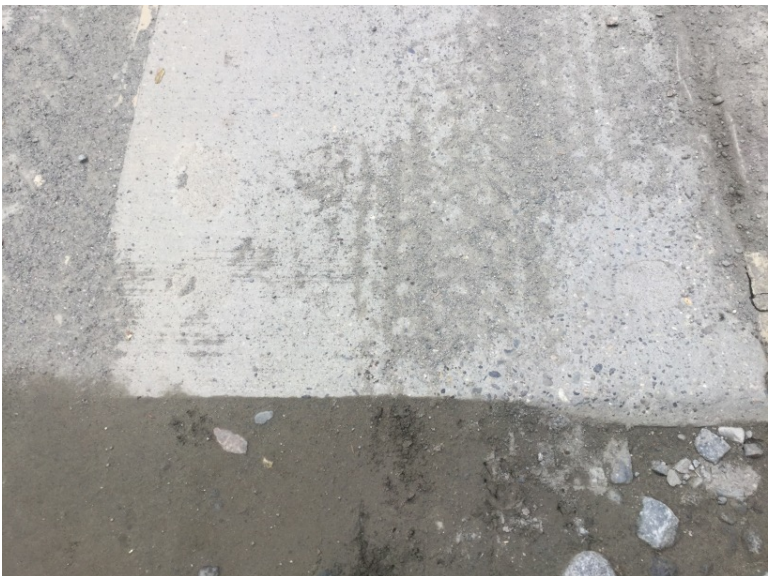
Each slab connected to cap in 2 locations at each abutment
