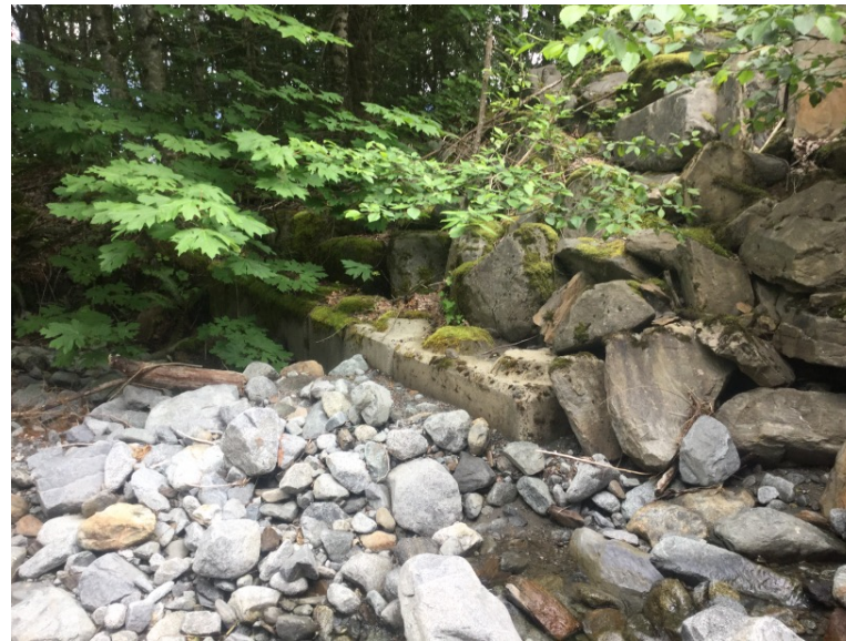
Lock blocks downstream right bank support riprap and fill
